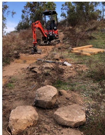
Work continues on the southern track Photo: Rob Lundie
